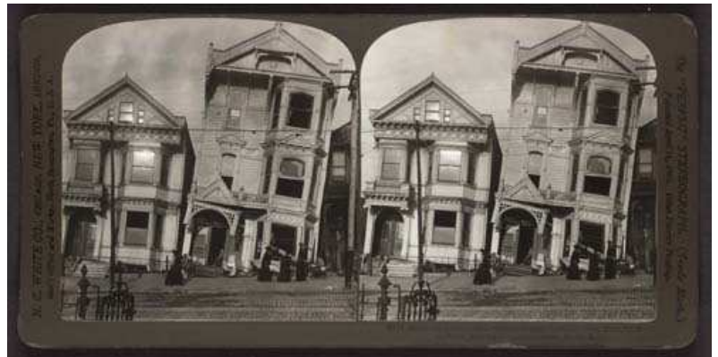
H.C. White Co., After the Earthquake—Frame Houses Tumbled from Their Foundations, San Francisco Disaster , 1906; stereoview; Prints and Photographs Division, Library of Congress, Washington, D.C.
